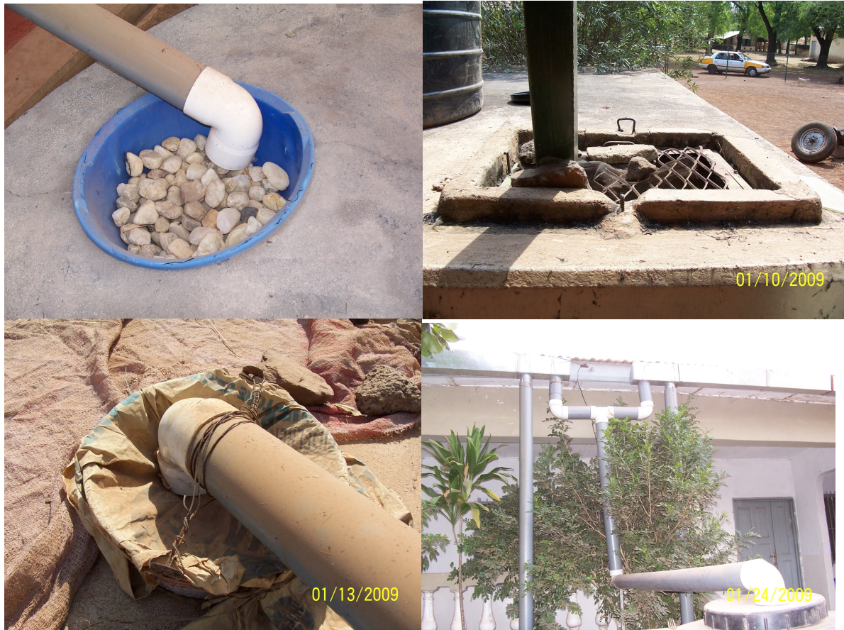
Figure 41: Examples of Storage Tank Inlets with Pre-filtering: Rough gravel in bucket pre-filter(upper left), degraded wire mesh partially covering inlet (upper right), cloth filter over gravel pre-filter(lower left), sealed tank entry after first flush with leaf screen (not visible) in guttering (lower right)
