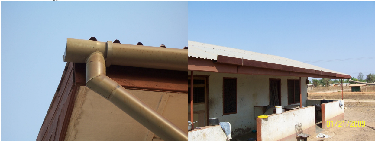
Figure 30: Custom-built gutter system fabricated in Accra using PVC pipe cut in half for gutter (left) and bent steel gutter fabricated by Fuseni gutter (right)
