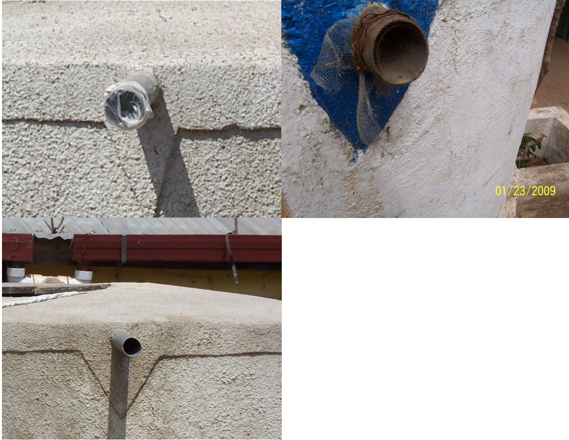
Figure 42: Overflow Pipes at Presbyterian Tank Program tanks: Covered (upper left), Screened (upper right) and Unscreened (lower left)
