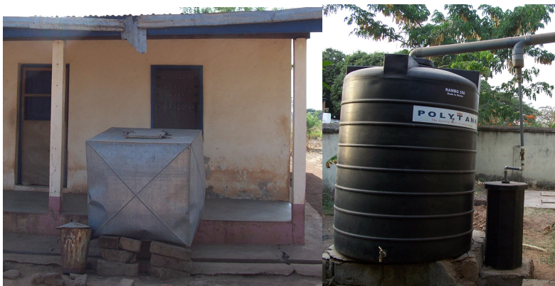
Figure 38: Foundation issues: Brick support at corners of storage tank causing structural damage and leaks, Pong-Tamale Health Clinic (left), cracked and broken foundation, PHW house (right)
