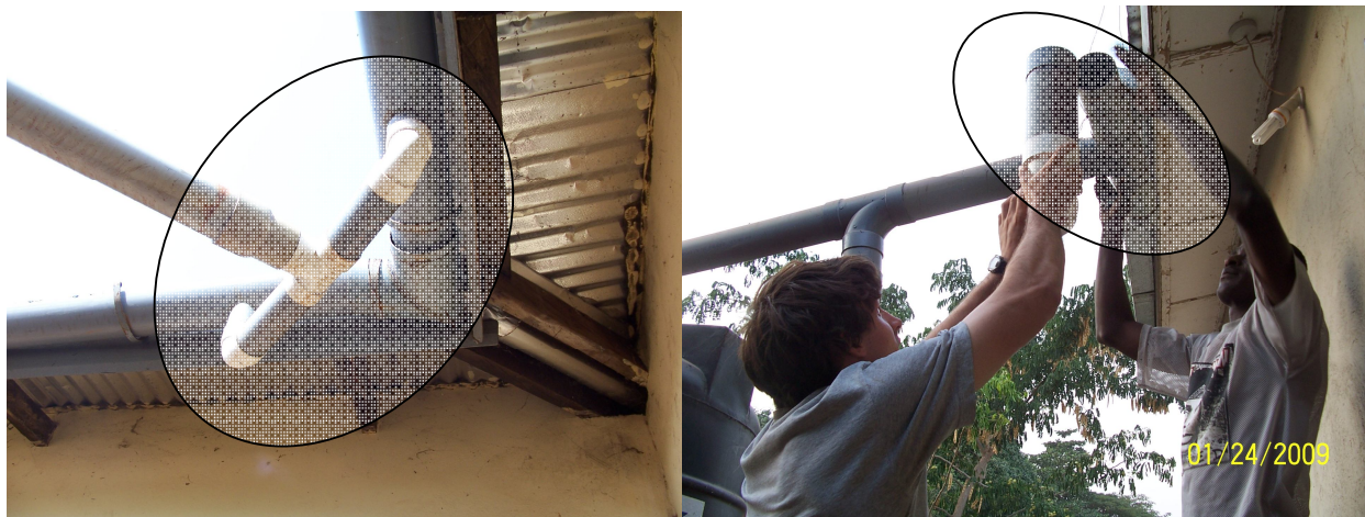
Figure 31: Leakage due to poor design (left) and author replacing sun-rotted PVC elbow joint at PHW house (right)
