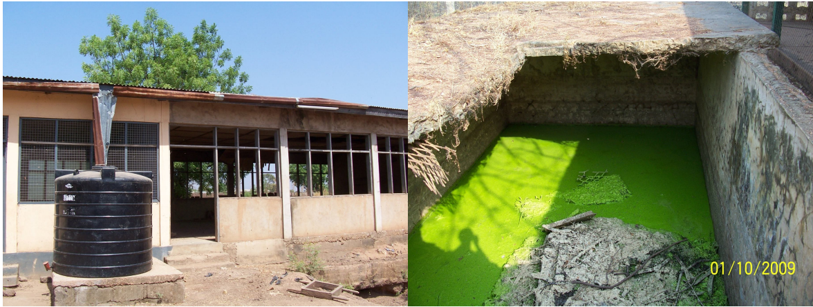
Figure 40: Durability: Unknown lifetime of plastic storage tank in full sunlight (left), structural failure of roof of subterranean reinforced concrete tanks, Veterinary college (right)
