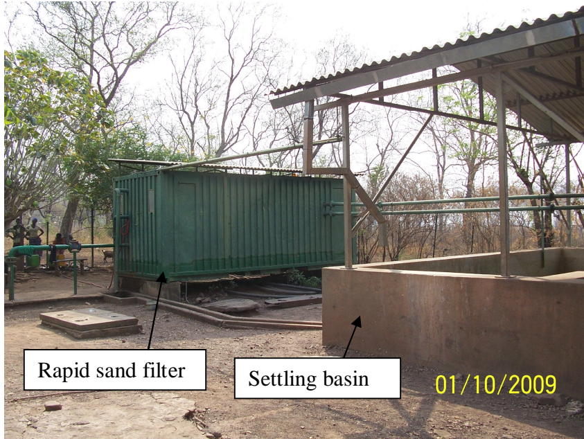
Figure 19: Treatment Facility at Veterinary College: Settling Basin (right) and rapid sand filter (trailer at left, see below)
