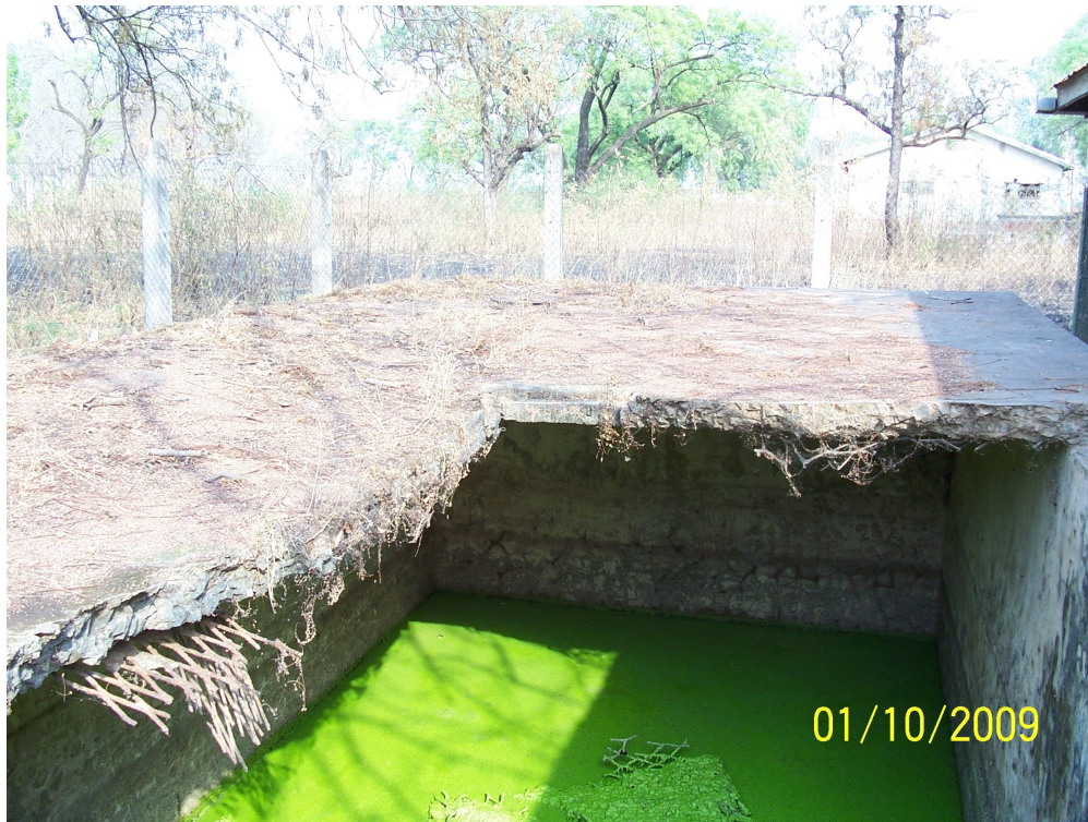
Figure 22: Underground storage tank on Veterinary College premises with collapsed roof
