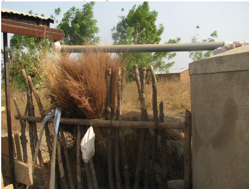
Figure 27: Manual first flush device: Removable Inlet Pipe (Photo Courtesy of Shanti Kleiman)
