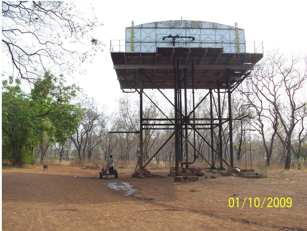
Figure 21: Storage Tank used for distribution to Veterinary College
