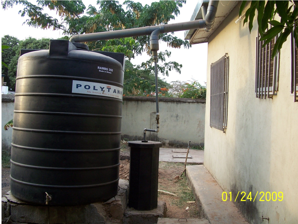
Figure 26: PHW RWH System in Rear of House
