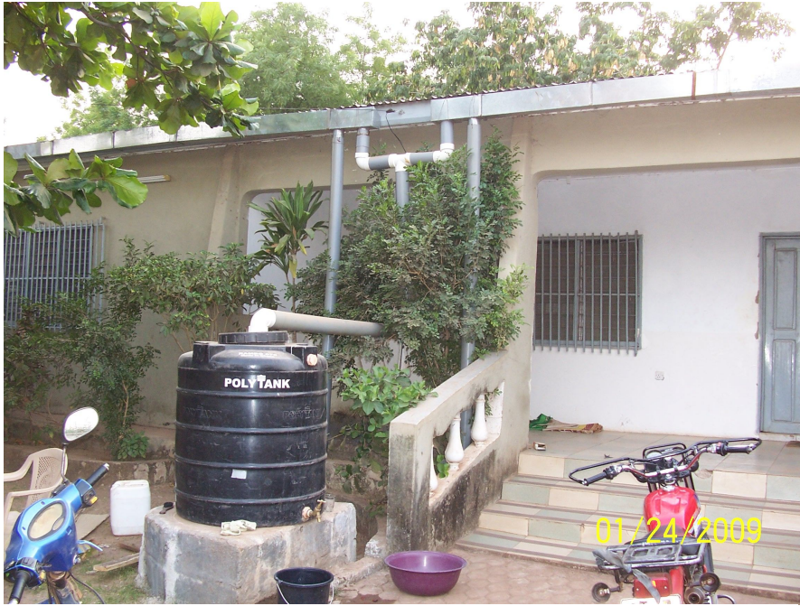
Figure 25: PHW RWH System in Front of House
