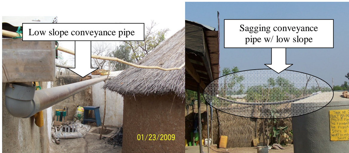
Figure 32: Low slope (left) of conveyance pipe to storage tank and sagging conveyance pipe with low slope (right)
