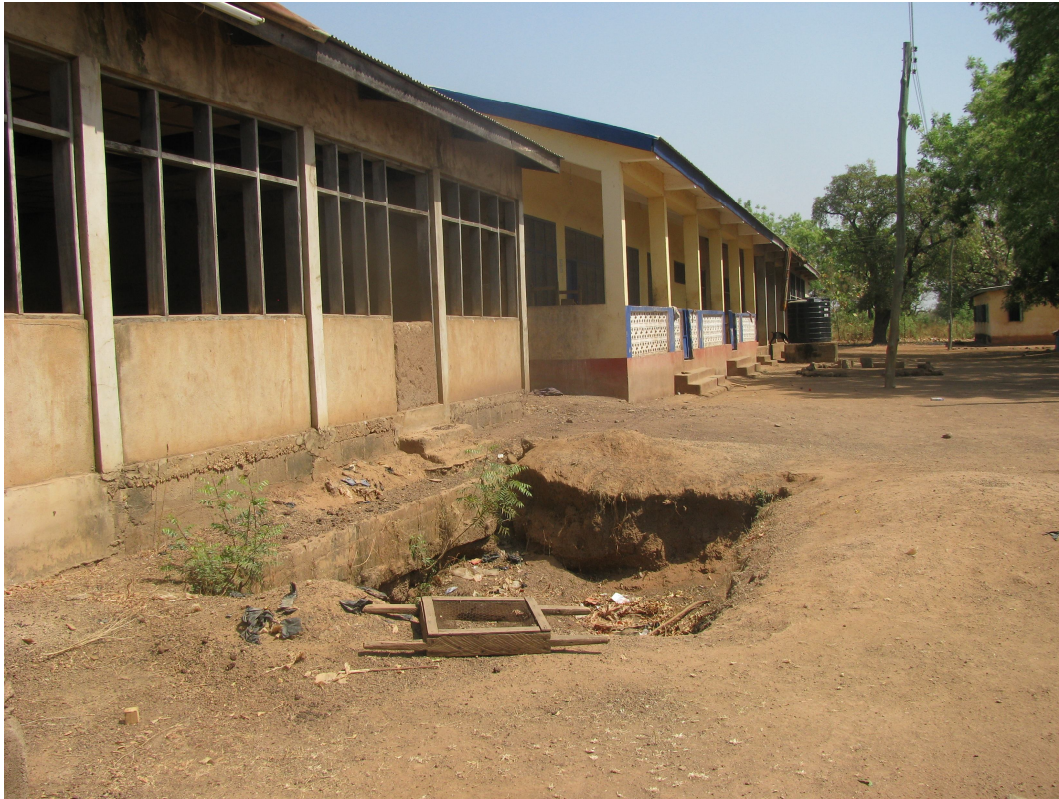
Figure 12: Pong Tamale Vocational School proposed site of underground storage tank
