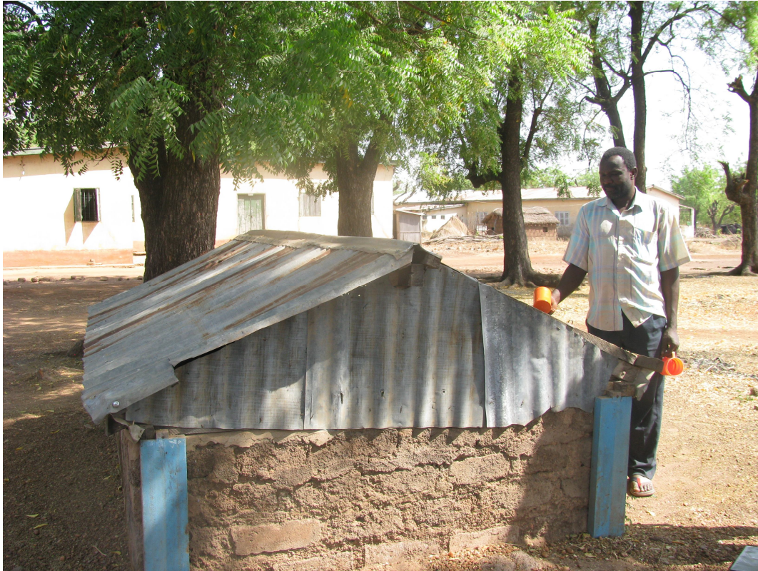
Figure 13: Pong Tamale Underground Storage: Water from tank used for bathing only
