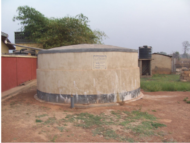
Figure 37: Leaky storage tank
