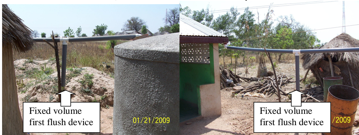
Figure 29: Fixed volume first flush devices: Presbyterian Tank Program
