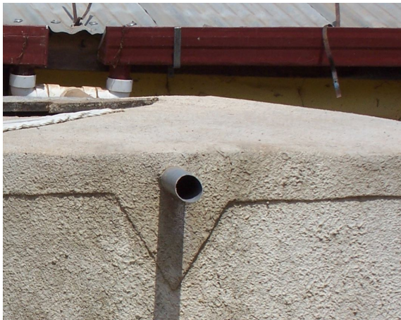
Figure 52: Unscreened Overflow Pipe
