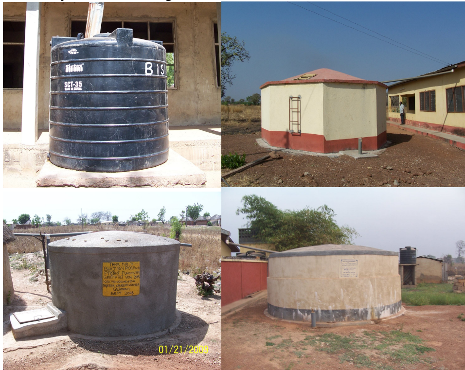
Figure 36: Four Different Storage Tanks: Plastic Storage Tank: Sintex Brand 1m 3 (upper left) Cement Block 75m 3 (upper right), Ferrocement 10m 3 (lower left), Cement Block 30m 3 (lower right)
