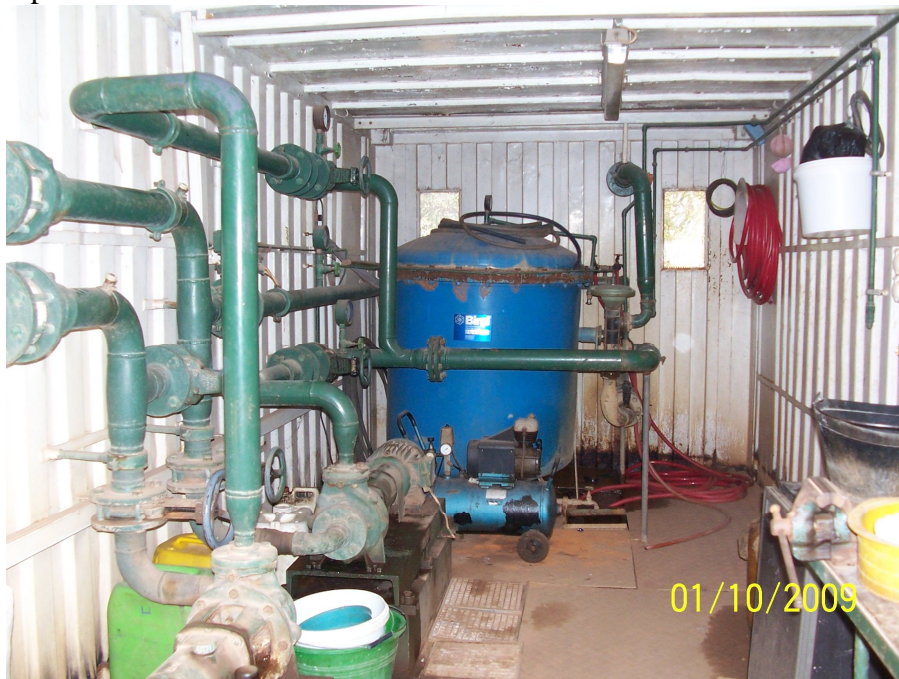
Figure 20: Rapid sand filter
